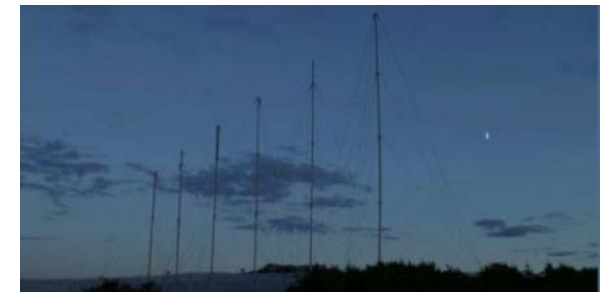
OTH RADAR ANTENNAS
